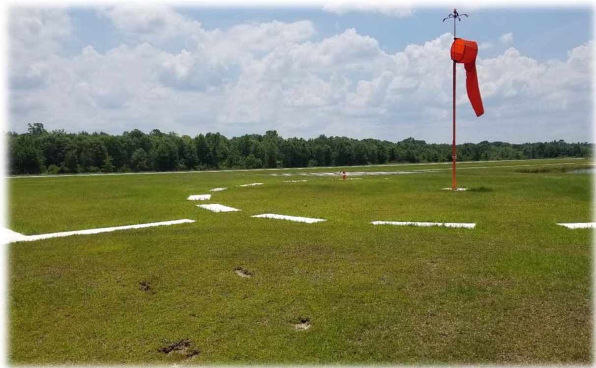
Figure 18: Existing L-807 Main Wind Cone with Segmented Circle (Centerfield)
