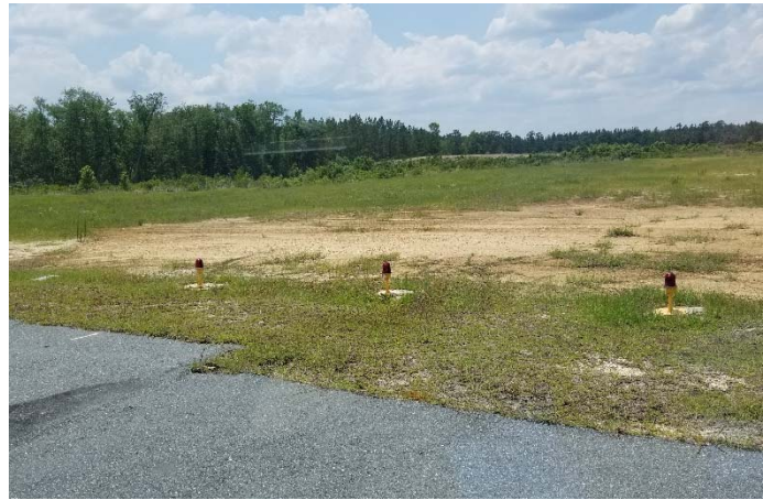
Figure 11: Runway Threshold Lighting
