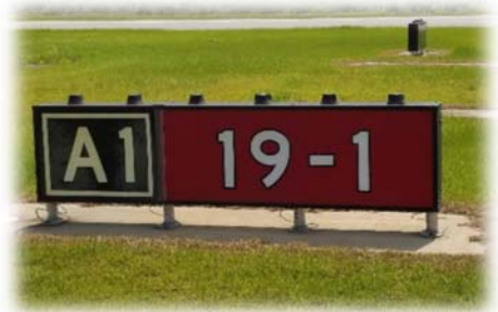
Figure 12: Taxiway Directional Sign and Mandatory Hold Sign
