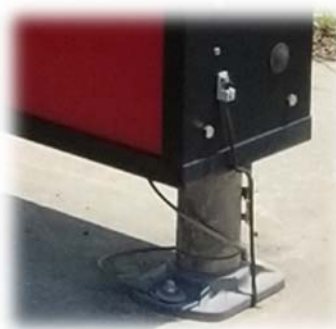
Figure 13: Sign Bonding to Ground Rod
