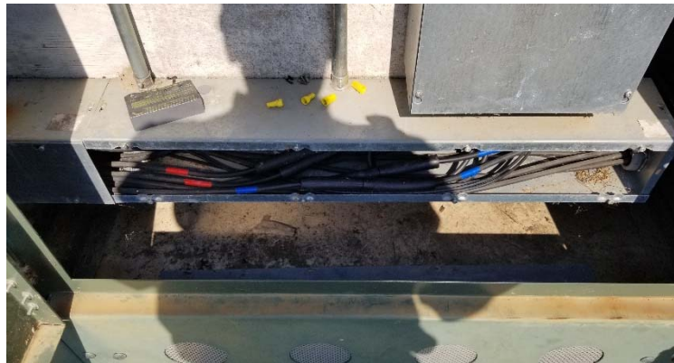
Figure 8: L-824 CCR Wireway
