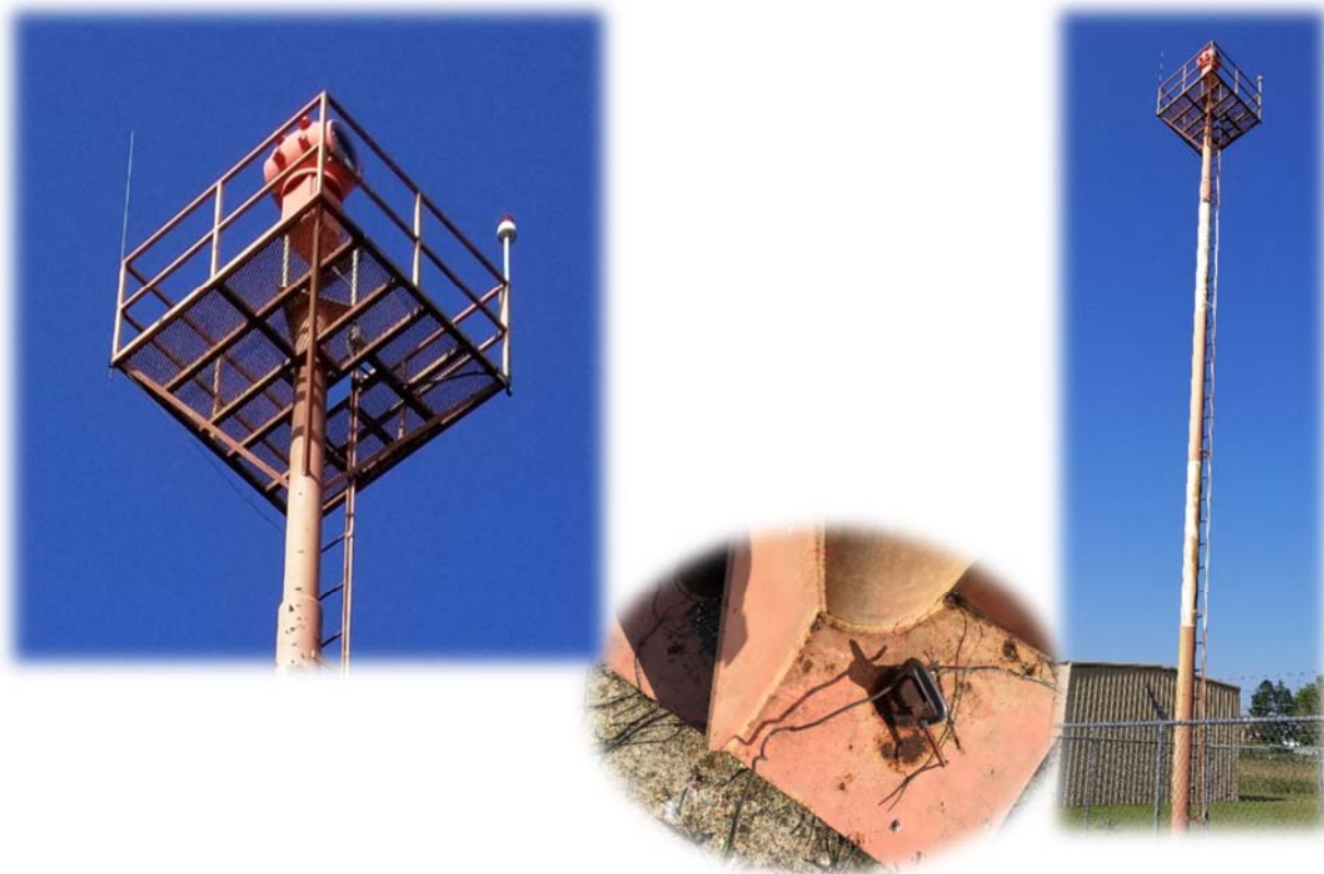
Figure 17: Airport Rotating Beacon and Tower
