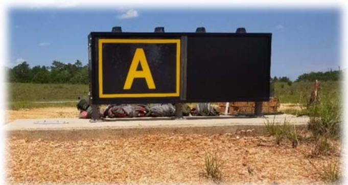
Figure 14: Sign Grade not in accordance with FAA EB 79
