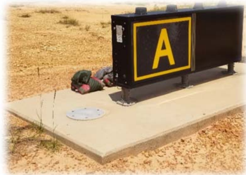
Figure 14: Sign Grade not in accordance with FAA EB 79
